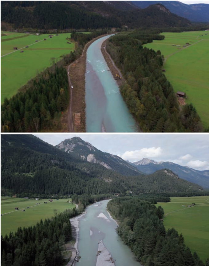
Figure 2 – Top: before restoration, bottom: after restoration. © Baubezirksamt Reutte
